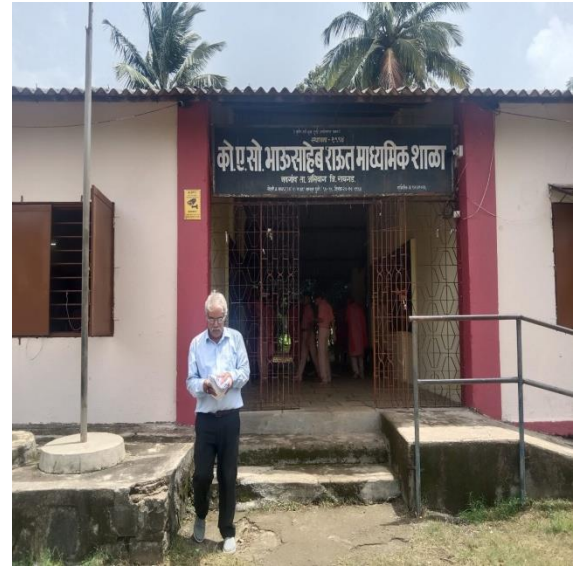
Painting and repairing work of Bhausaheb Raut Madhyamik Shala
